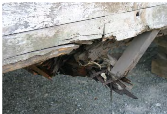
Areas of structural deterioration in support beams under the cabin.
