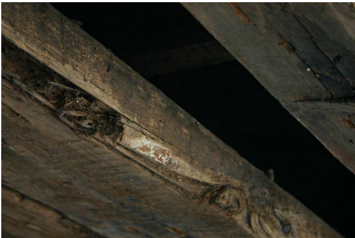
Detail of brown cuboidal fungal deterioration, frass& small flight holes of insects, possibly furniture beetle or carpenter ant.
