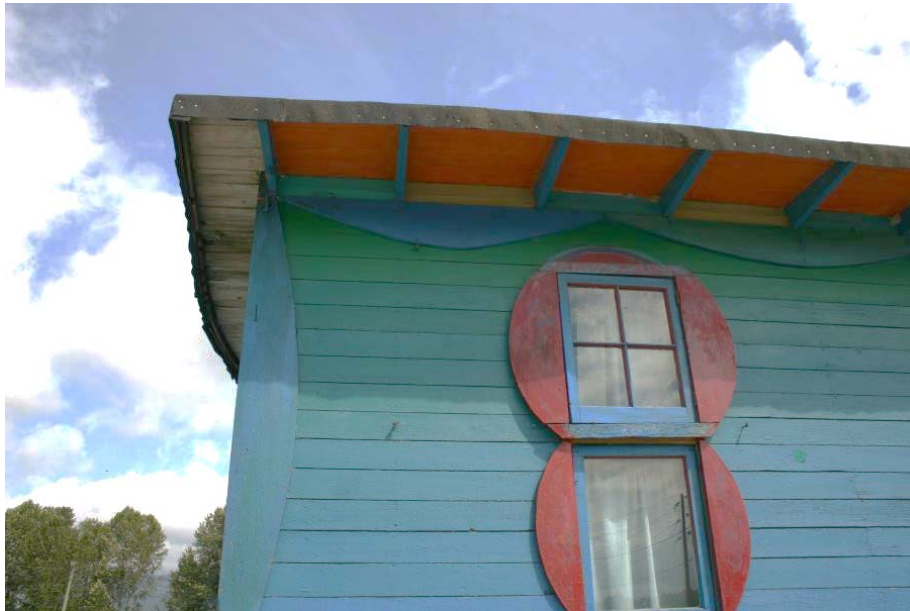
Detail of scalloped decoration and decorative finishing of the underside of the eaves. (Andrew Todd)
