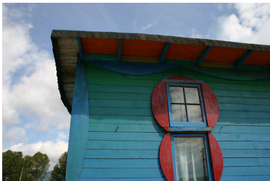
Detail of scalloped decoration and decorative finishing of the underside of the eaves.
