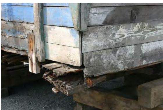
Areas of structural deterioration in support beams under the cabin.
